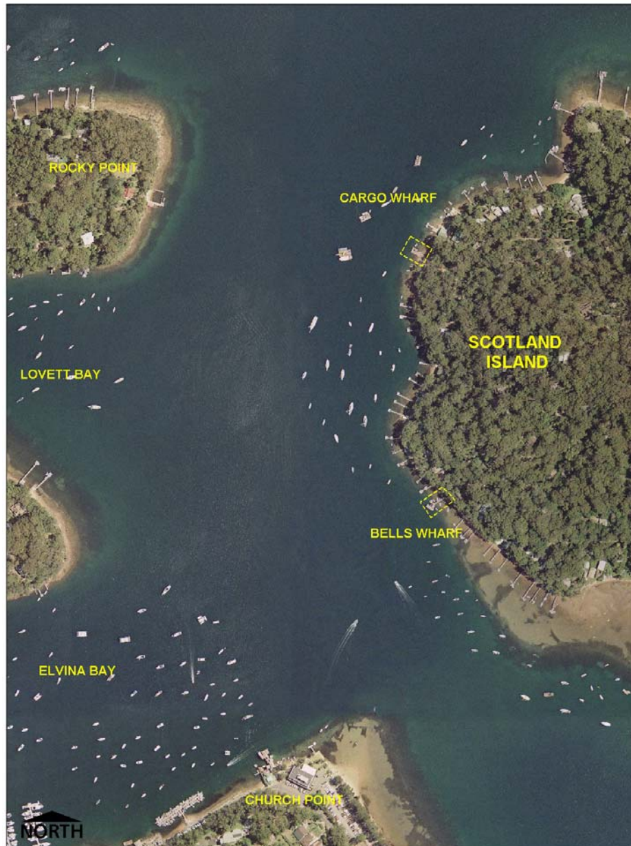
Aerial photography - Jan 2005 (Licensed from Sinclair Knight Merz.) This plan is not survey accurate.
