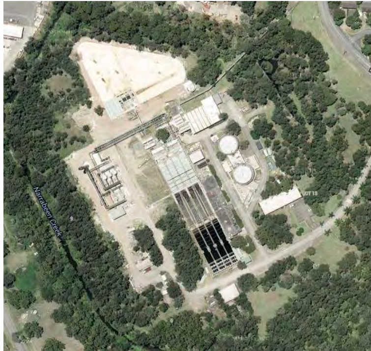
Figure 1: Warriewood STP before recent upgrades.
