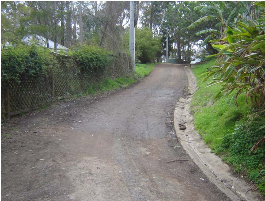
Plate 2 – View East on Florence Street (note crushed concrete dish drain)
