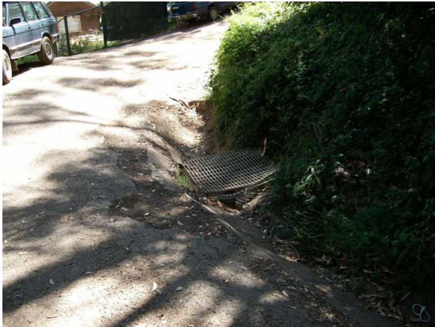
Plate 20 - Damaged pit grate at bottom of Harold St
