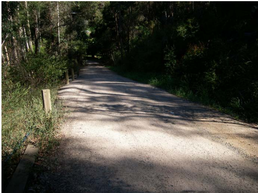
Plate 48 - Resin sealed section of Rd behind Catherine Park
