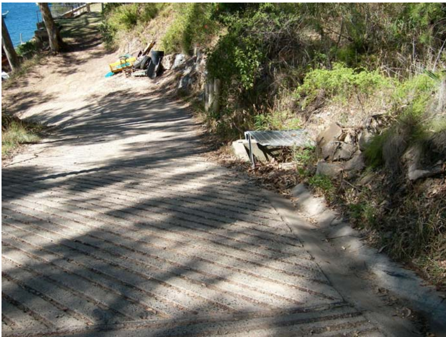
Plate 36 - Concrete dish drain and pit on Cargo Wharf Rd
