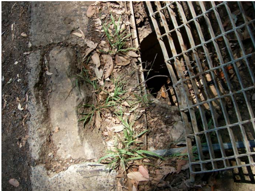
Plate 20 - Damaged pit grate at bottom of Harold St
