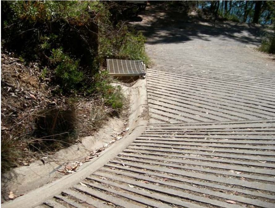
Plate 36 - Concrete dish drain and pit on Cargo Wharf Rd
