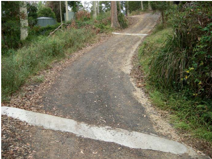
Plate 70 - Thompson St just past int. with Harold ( note concrete water bars )
