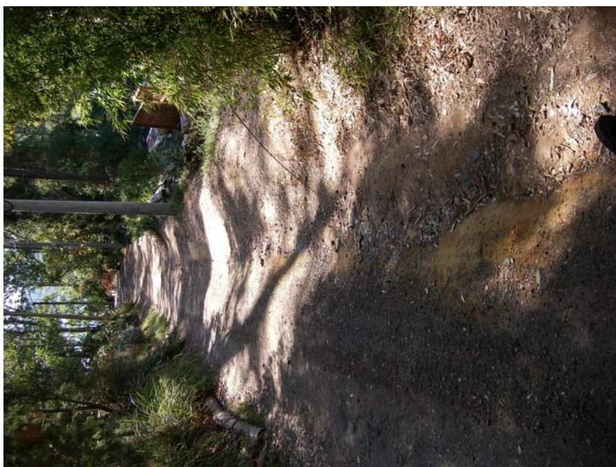
Plate 46 - Eroded section of Robertson Rd
