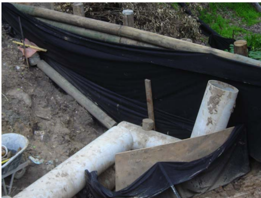
Plate 10 - Construction of new culvert under Richard Road at landslide site
