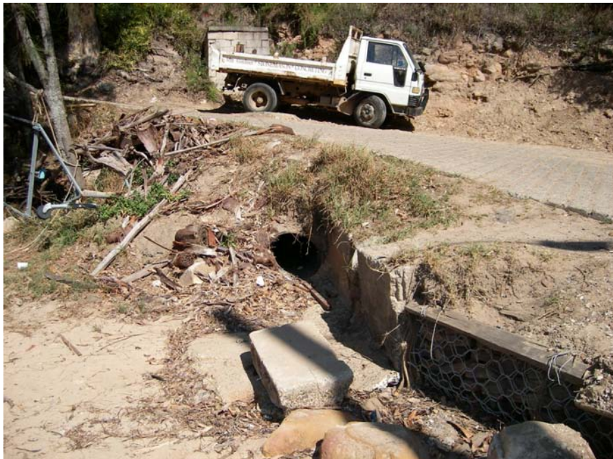
Plate 38 – Stormwater outlet at Cargo Wharf
