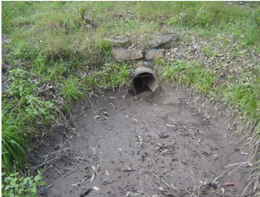
Plate 4 – Existing Sediment Basin at Stormwater Outlet into Catherine Park
