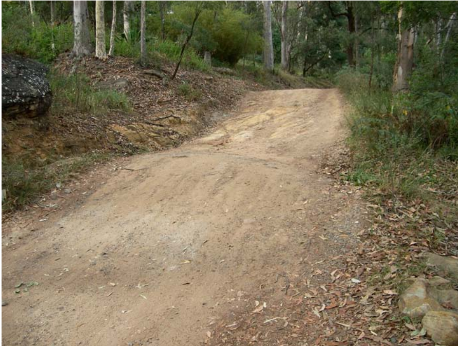
Plate 60 - Outlet of Waterbar from Plate 59
