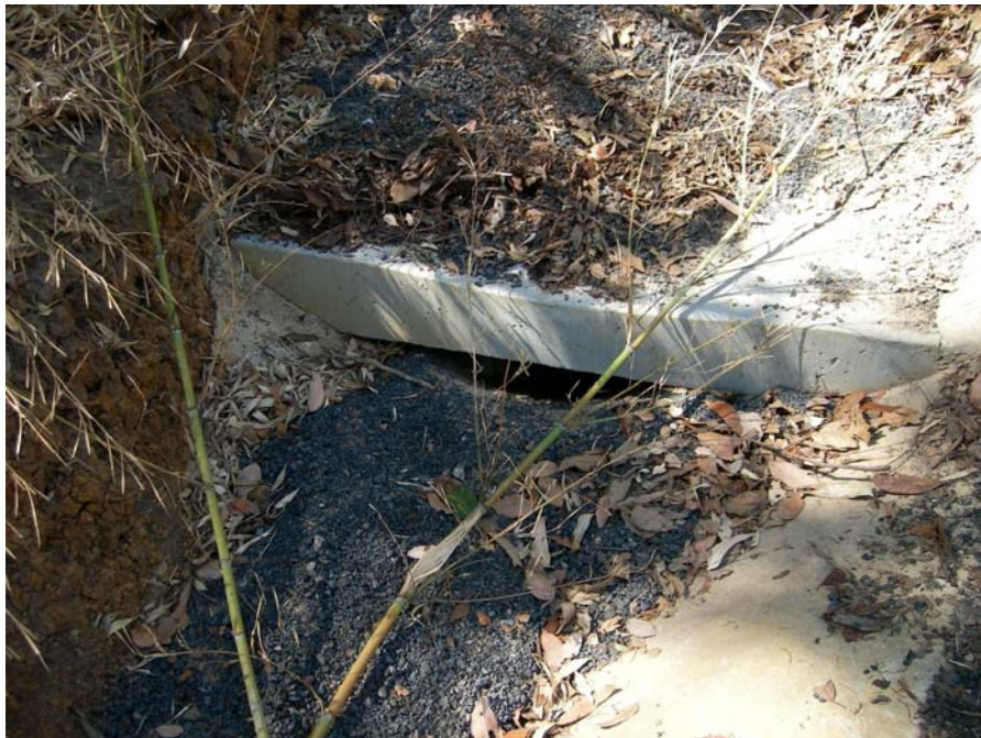
Plate 22 - Blocked pit at int. of Richard Rd and Cecil St
