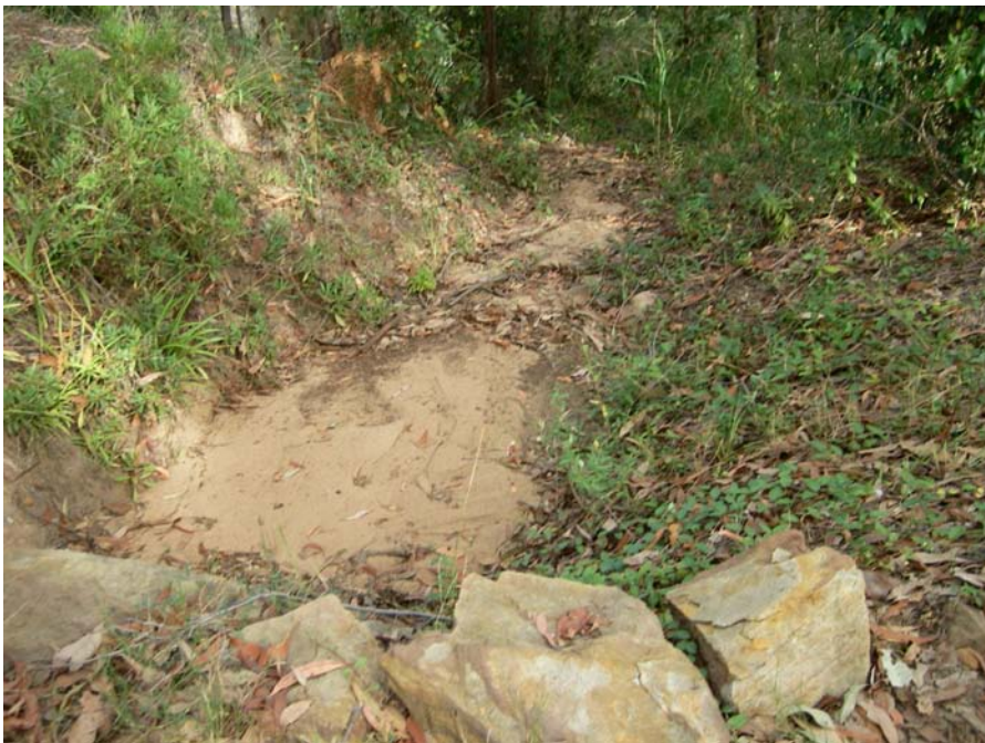
Plate 60 - Outlet of Waterbar from Plate 59
