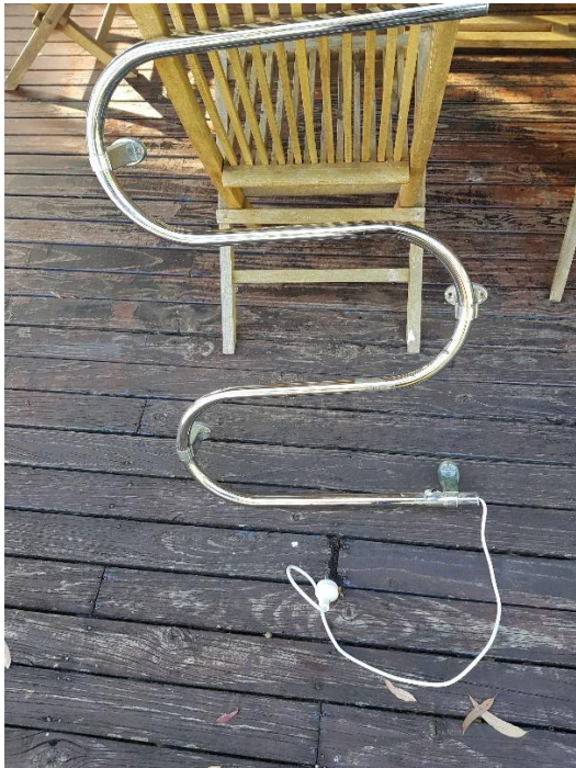
Heated towel rail. Some surface rust but operational prior to decommissioning.
